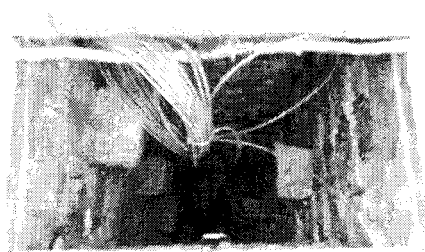
Fig. 11.2(e) Dug well (lined with stone blocks).
