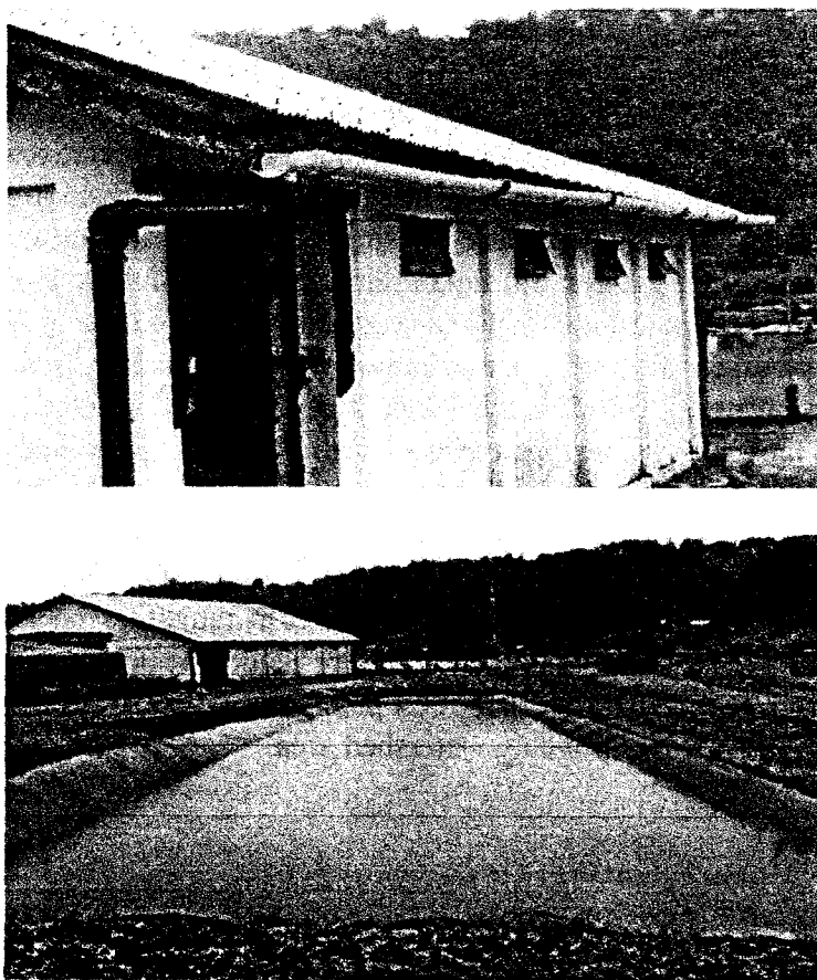
Fig 3. Roof water harvesting in Silpaulin lined pond at ICAR, Umiam, Meghalaya.
